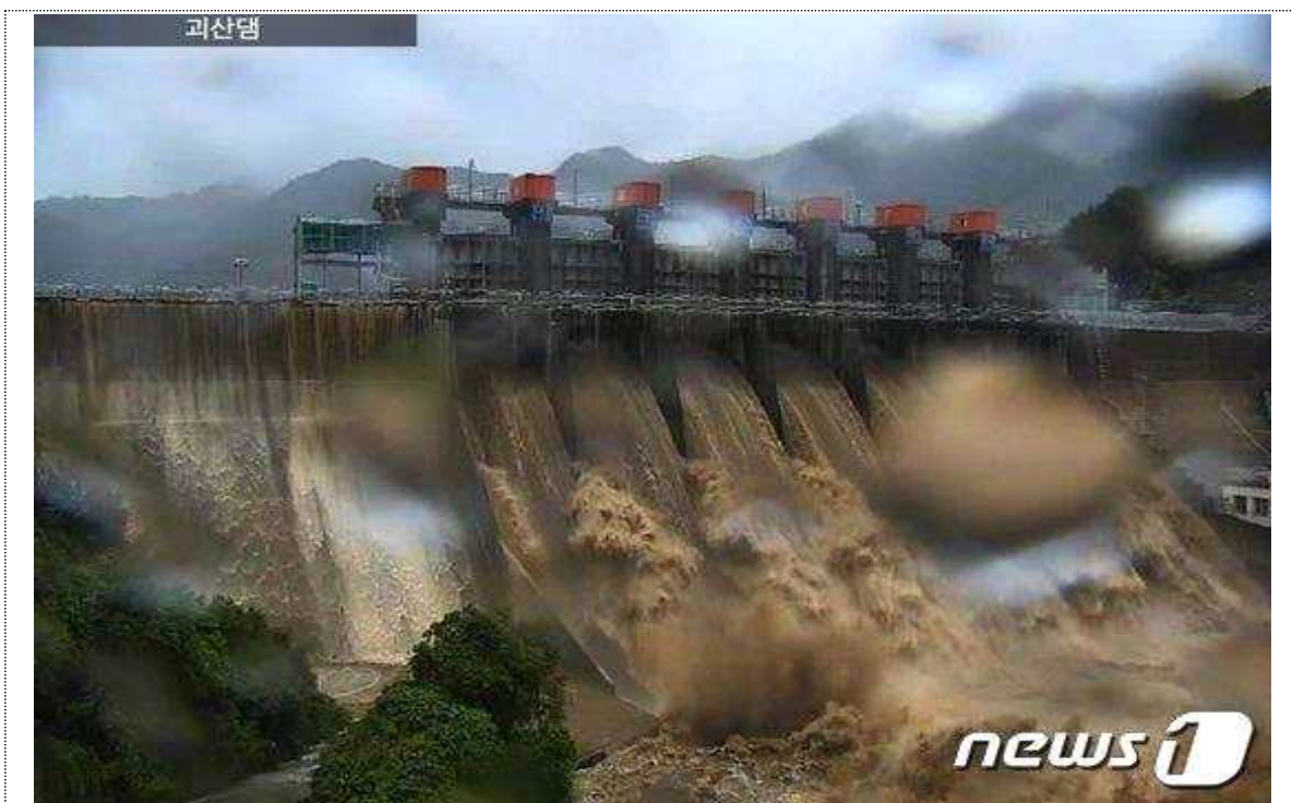
Figure 6 Photo of Goesan Dam overflow discharge
