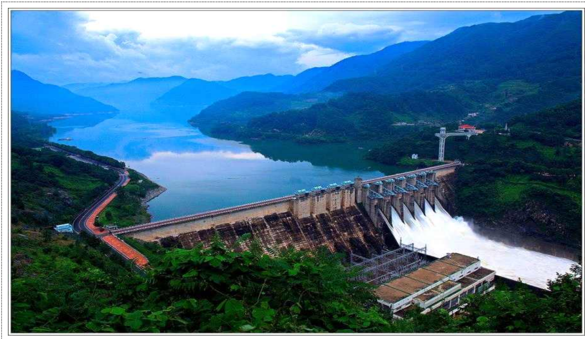
Figure 1 Chungju Dam Site Photo
