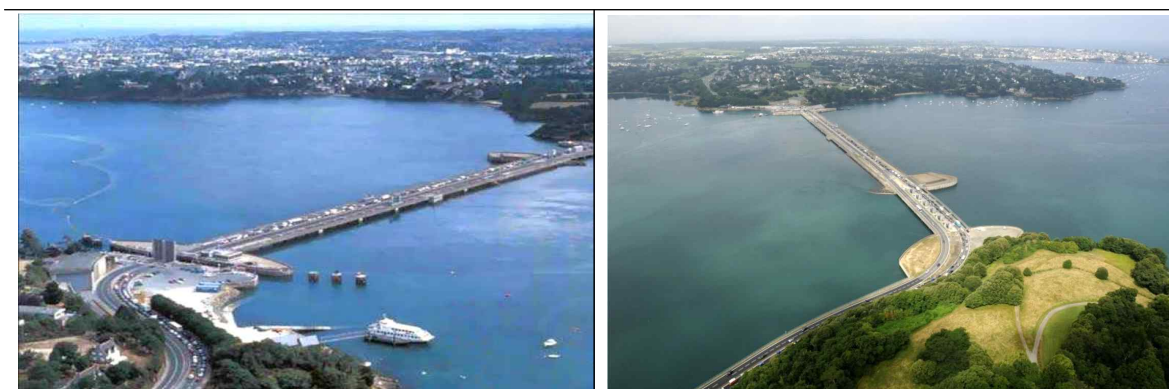
Figure 3. Rance Tidal Power Plant in France
