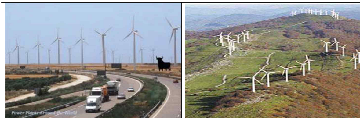
Figure 2. Wind farm in La Muela, Navarre
