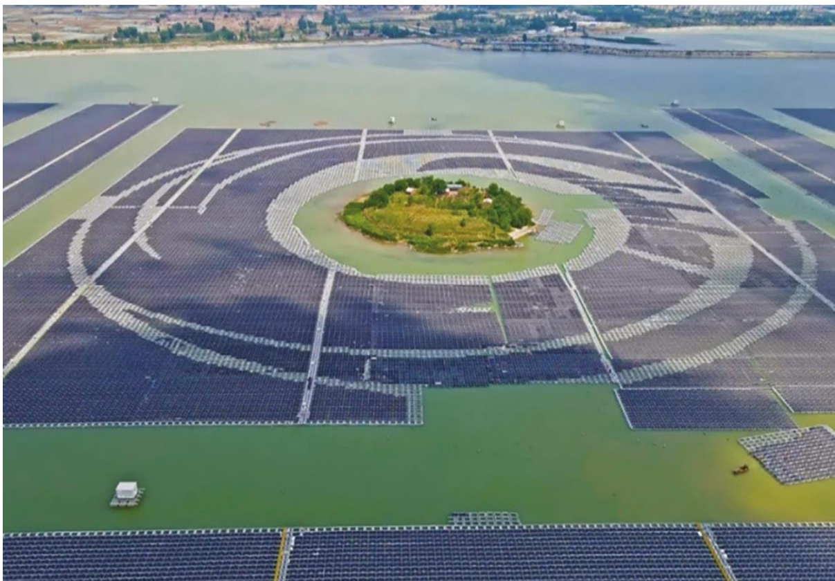
Figure 5. floating photovoltaic power plant in china
