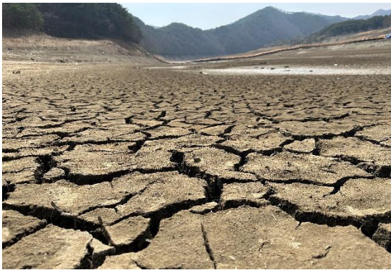
Floor View of Juam Dam Due to Drought
