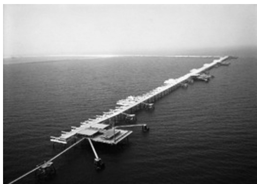
Figure 2-8 | Jubail Port Construction Project
