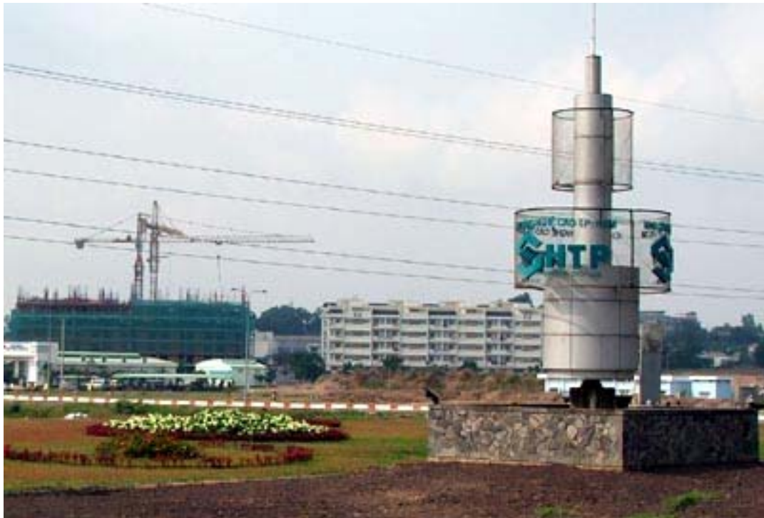
Figure 31 Defects occur during the execution of SHTP
